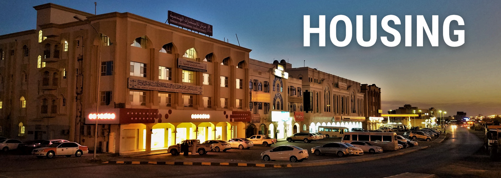
Typical apartments in Oman
